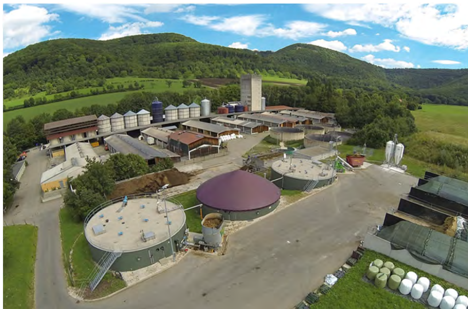
Research biogas plant on a practical scale at the Unterer Lindenhof with post digester (center, integrated gas storage) and two identical digesters (concrete roof with sampling ports)
