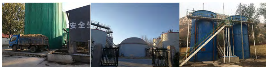
The three plants of the Chinese biogas measurement program (October 2017)
