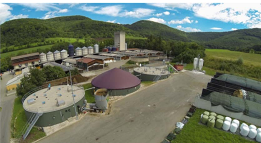
Research biogas plant digesters with mechanical substrate pretreatment
