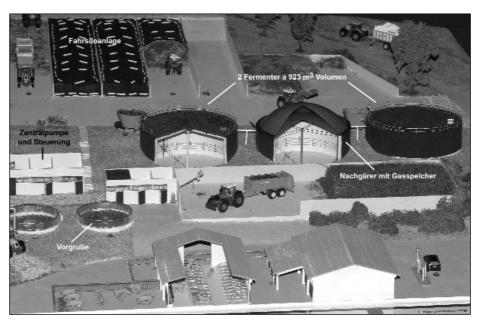
Fig. 1: Design model of the research biogas plant "Unterer Lindenhof"
