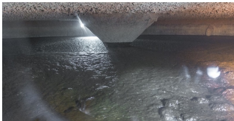
The biogas composition will be measured directly in the digester in order to be able to react to process disturbances at an early stage (2018, University of Hohenheim)
