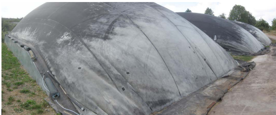
Solids fermentation plant (Pertagnol, 2019)
