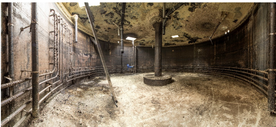
Modification measures in the fermenter of the research biogas plant for sensor-based detection of the stirring requirement (2021, University of Hohenheim).
